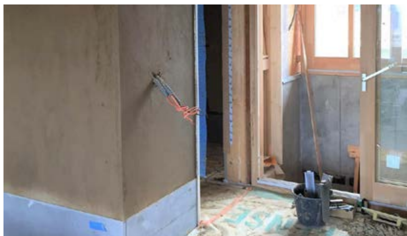
Finitions intérieures (@ designbuildLAB, ENSAG)
