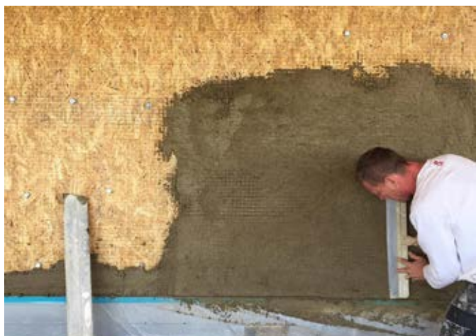
Finitions intérieures (@ designbuildLAB, ENSAG)
