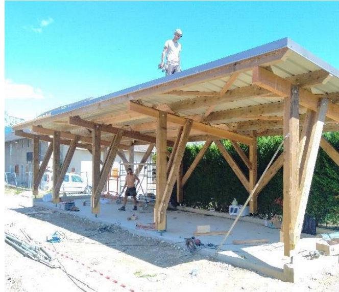
Installation abri vélos
